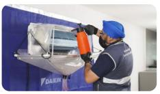
Alkaline-based chemical will be applied on the coil to wash off dirts and bacterias.
