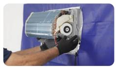
After covering the surroundings, technician will start to dismantle the air filter, casing, blower and control box.
