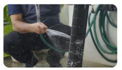
The air filter, casing and blowers will be washed externally.
