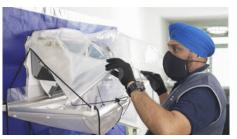
After dismantling, technician will hang a cover over the aircond.
